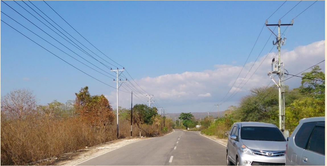
Road, Electricity, Telephone and Internet Networks
