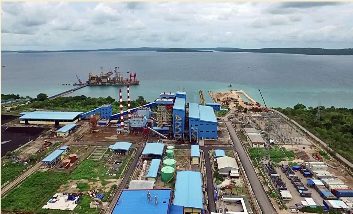
PLTU BOLOK (Power Plant with a capacity of 73 MW)
