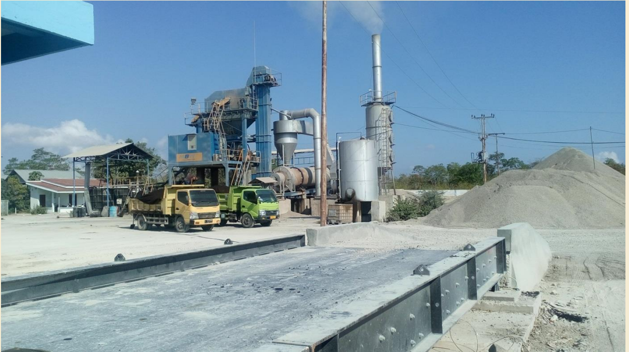
PT. Dwi Sejati Beton (Ready Mix)
